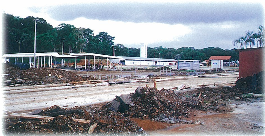
Fort Davis Export Processing Zone project, Panama.
