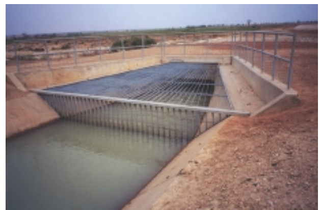
▲ Bagre Right Bank Farmland Reverse Siphon Construction
