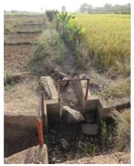
Figure 13. Deterioration of irrigation facilities
