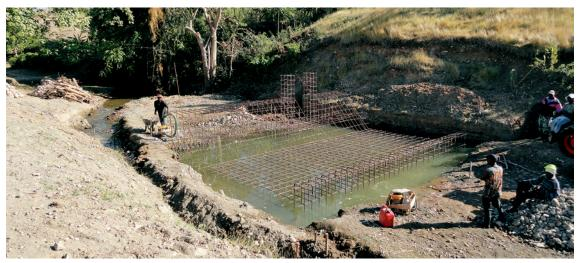
Through its humanitarian assistance operations, the TaiwanlCDF has been assisting in Haiti's post-disaster recovery following the recent major earthquake. Shown here, engineering work for the construction of a weir as part of the New Hope Village Water Supply System Project.
