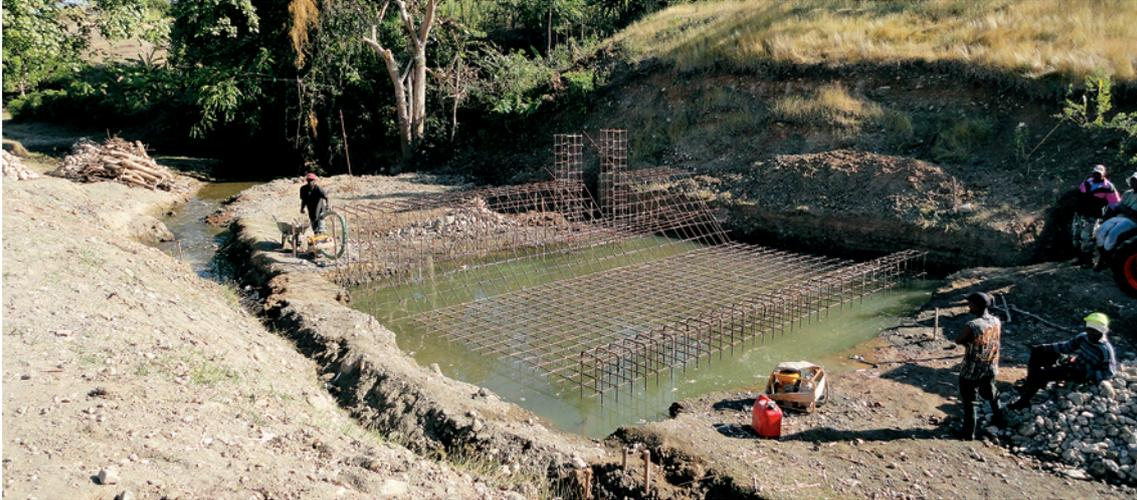
Through its humanitarian assistance operations, the TaiwanICDF has been assisting in Haiti's post-disaster recovery following the recent major earthquake. Shown here, engineering work for the construction of a weir as part of the New Hope Village Water Supply System Project.
