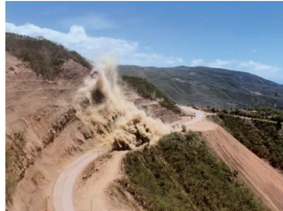
The photo shows the mountain blasting work in phase three of the Guatemala CA-9 Highway Construction Project.
