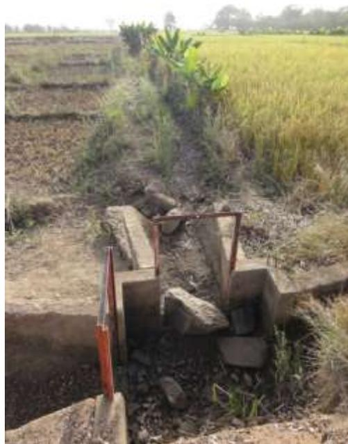
**Figure 13.** Deterioration of irrigation facilities
